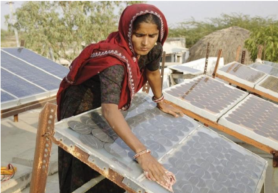
An Indian villager works on a typical solar photovoltaic installation.
